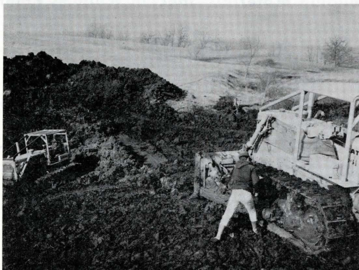
Chuck Allgood, Conservation contractor, is shown digging the core trench for the large livestock water and recreation pond on the Earl Edwards farm in Pleasant Grove twp.
