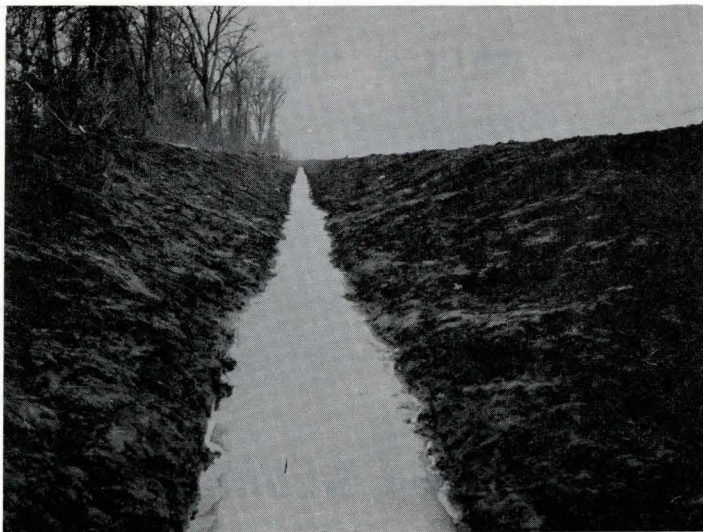
Sam Stonoff of Huron Twp. completed this 2,300 ft. long open drainage ditch late last winter. This ditch will provide surface drainage and intercept some of the seepage water from the Mississippi River.
