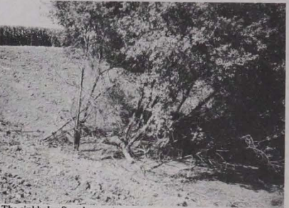
The sinkhole after clean out.
