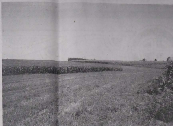
The grassed waterway at the Kathryn Hinsenbrock farm North of West Union is properly maintained. The waterway has an adequate width which helps it convey runoff during heavy rainstorms. (SWCD file photo)
