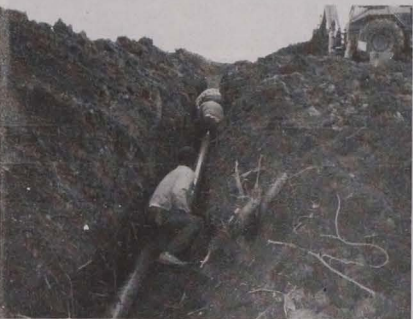
Contractors laying plastic pipe used as principal spillway on the Ridenour farm.
