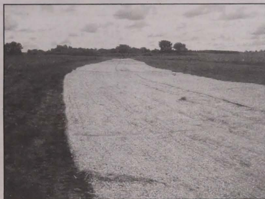
Newly constructed and seeded waterway with installation of a mulch blanket for erosion control.
