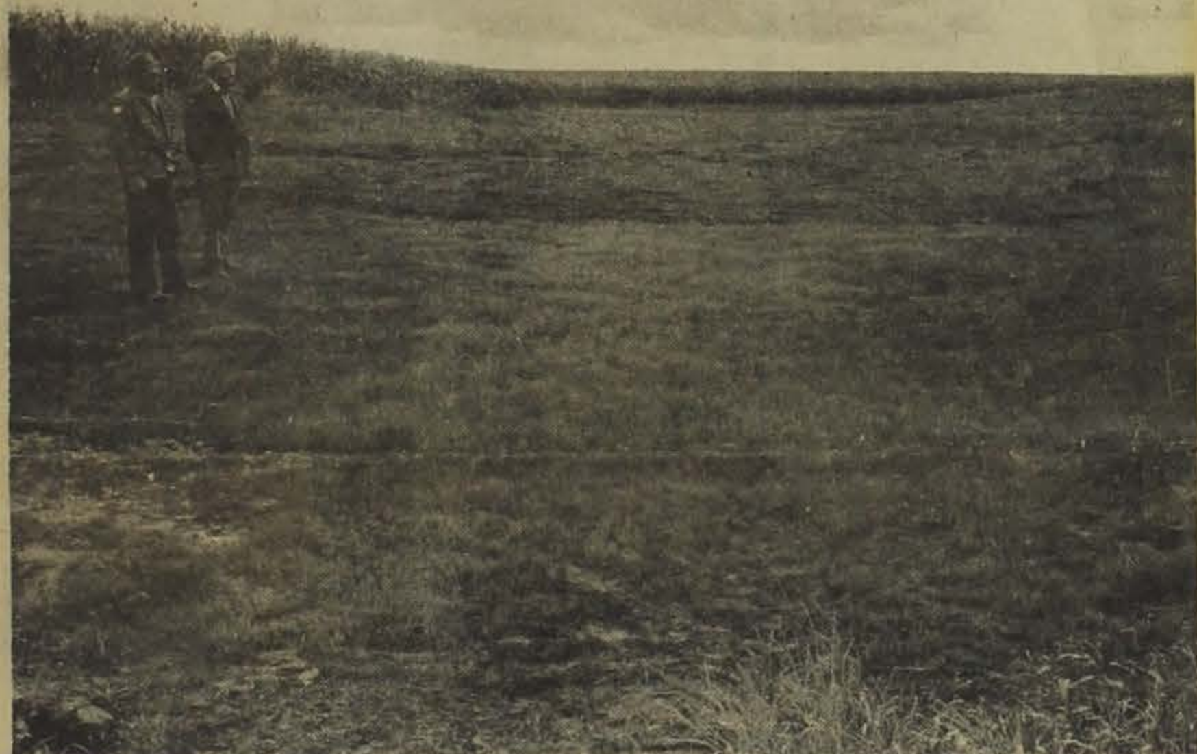
Left to right are Larry Holst and Hank Kavalier looking at the newly seeded waterway which is also protected by a mulch material called Enkammat. The use of the Enkammat will replace a concrete structure at this waterway outlet and will only cost one-fourth as much.
