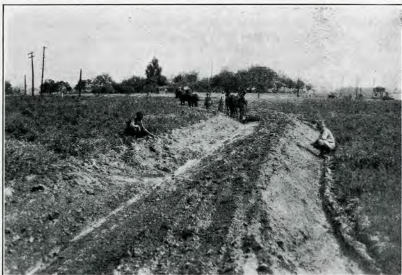
FIGURE 19.—Terrace construction with the plow and V-drag. It requires considerable work to develop satisfactory terraces with this type of equipment.
