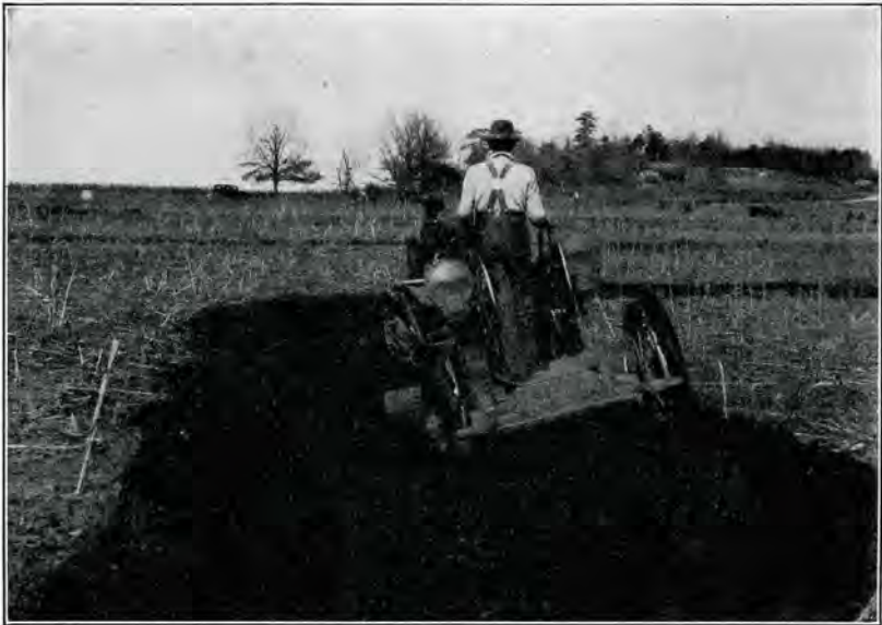
FIGURE 21.—Terracing with a 10-foot blade terracer and crawler-type tractor. This type of equipment is used extensively for terrace construction.
