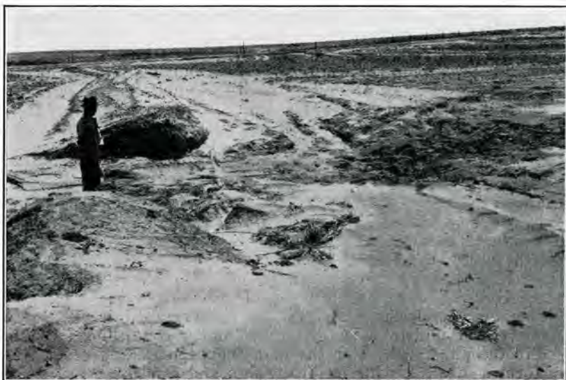
FIGURE 8.—Overtopping, caused by improper design, construction, or maintenance of terraces, damages both field and terrace.
