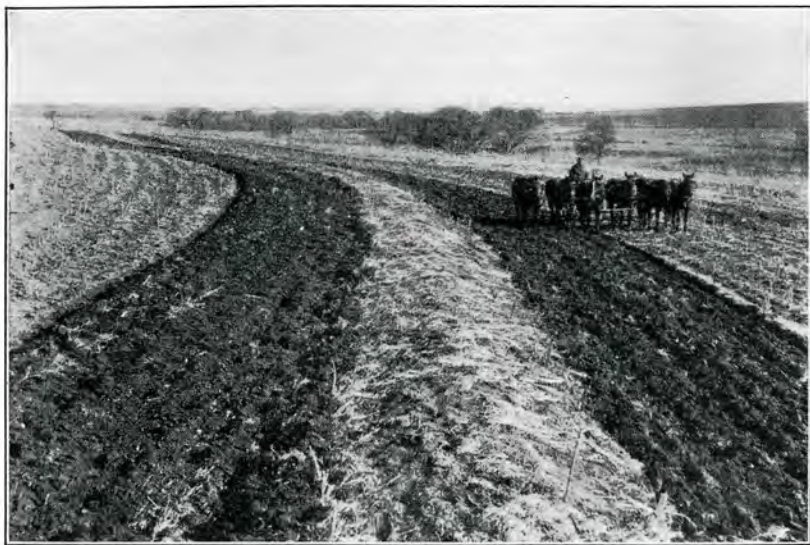
FIGURE 30.—A terrace ridge can be made wider and the side slopes reduced by backfurrowing toward the ridge.
