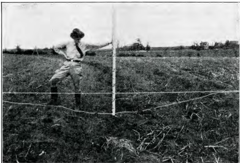
FIGURE 10.—The drainage-type terrace in the Piedmont area. It is important that a wide channel with ample capacity be provided.
