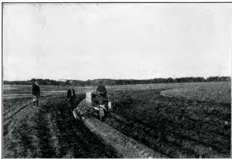
FIGURE 31.—Plowing a drainage-type terrace in order to maintain proper cross section. Note how the channel is being plowed out and how the terrace has been blended into the lower slope.
