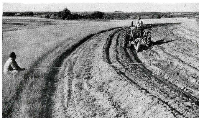
Plowing out the channel of a terrace. Lines indicate cross-section of terrace.
