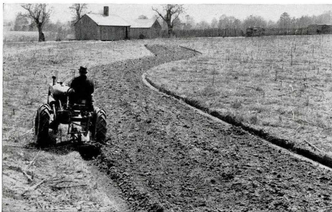
Building a terrace with a turning plow.
