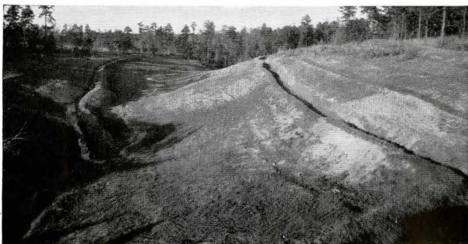
Controlled slope diversion ditches built to permit healing the gullies shown in the foregoing picture.
