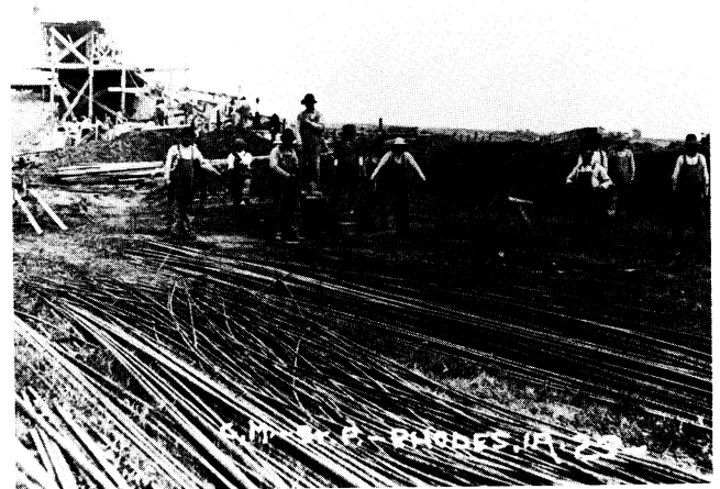
Construction of the Chicago, Milwaukee and St. Paul Bridge west of Rhodes.
