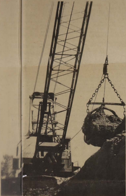
Digging the first cut
