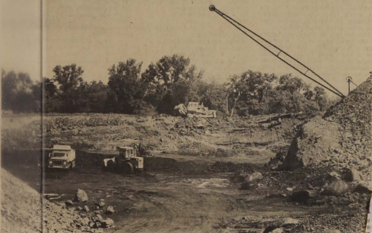
Strip pit is scene of several operations
