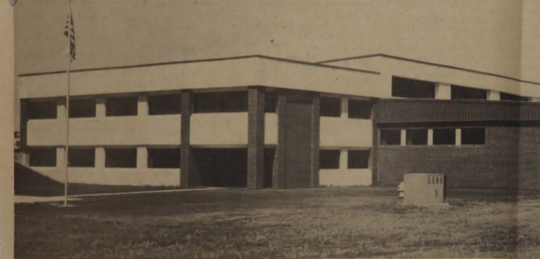
Water treatment plant at Rathbun.
