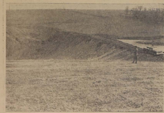
As Work Was Starting
