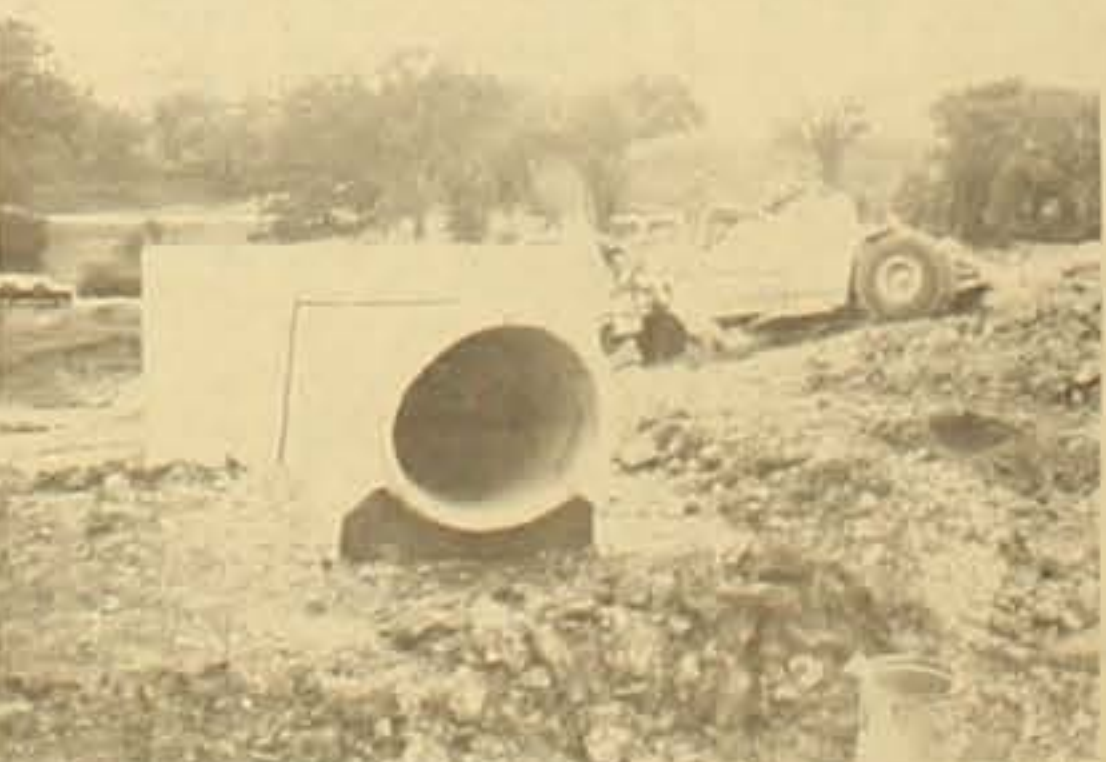
Construction of the dam at the East Lake of Osceola was completed last fall. As part of the RC&D project, the outlet pipe is shown during
