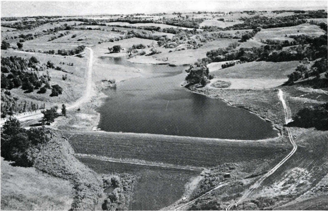
STRUCTURE SITE NO. 30 - PONY CREEK WATERSHED - 2 MILES WEST OF GLENWOOD.
