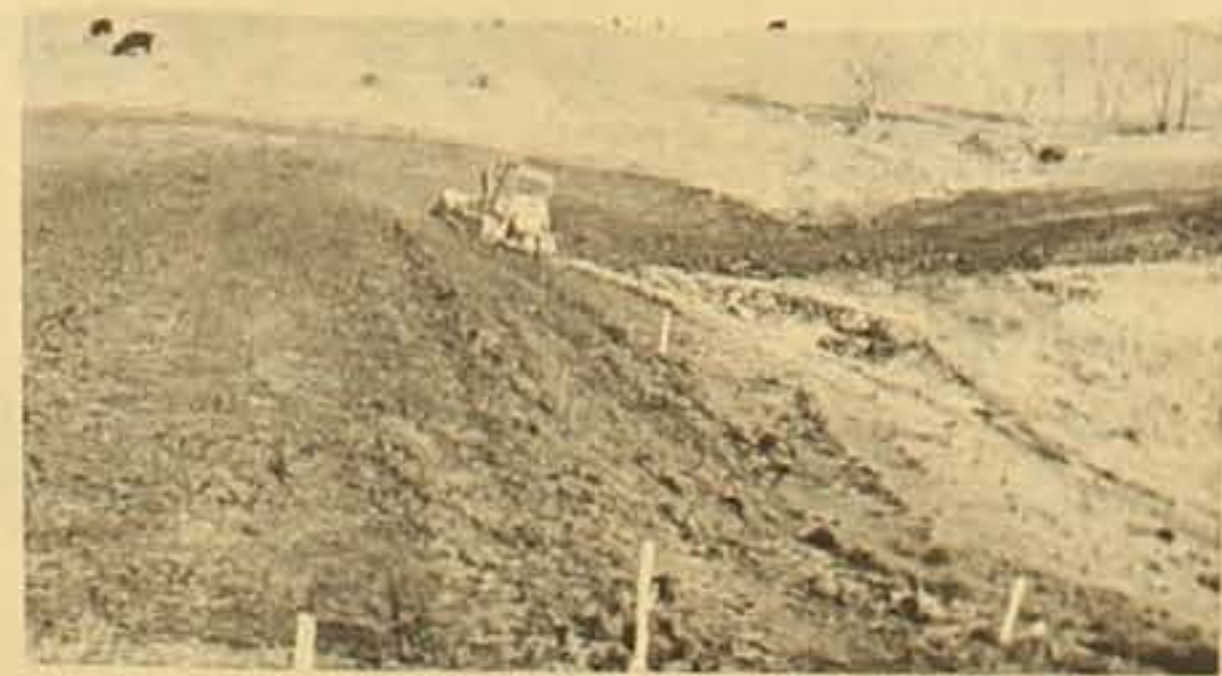
Approximately 10,000 cubic yards of dirt are now in place, making up the dam that will create a 1.5 acre pond. Funds, in the amount
