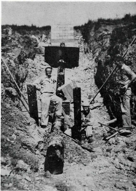
Installation of the pipe on the Lauder farm in the same location of the gully head in previous or above picture. This picture shows the cement block riser, metal cut off wall or anti-seep collar and the post for the propped outlet.
