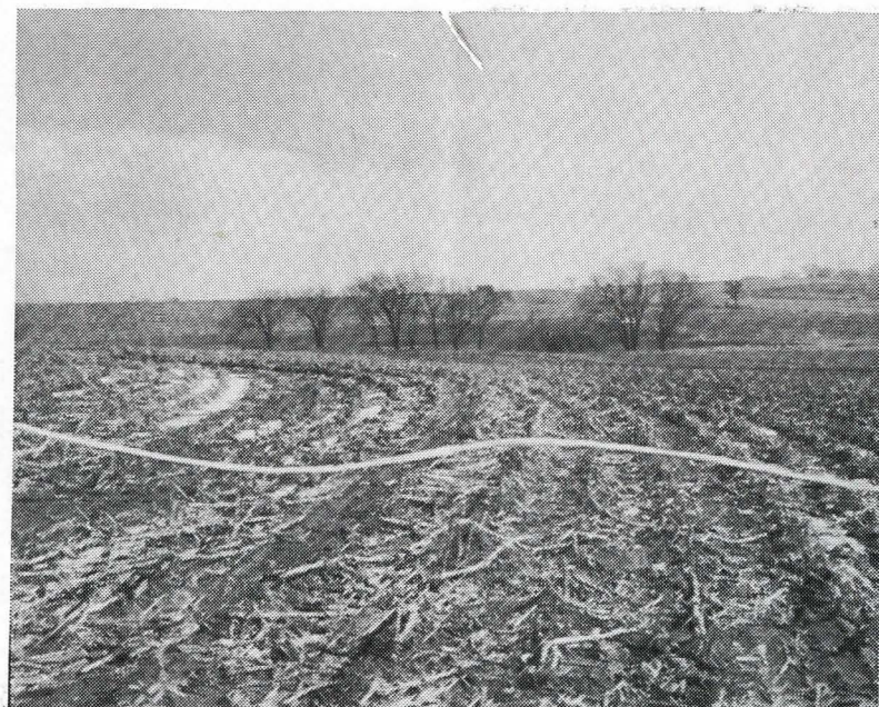
A broad base terrace is designed to fit modern farm machinery. Notice the number of corn rows on these slopes.
