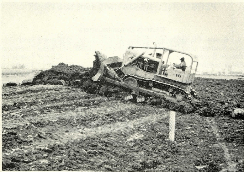
Parallel tile outlet terrace under construction on Warren Claney farm. Terraces do an effective job of controlling water runoff and keeping soil on the farm.
