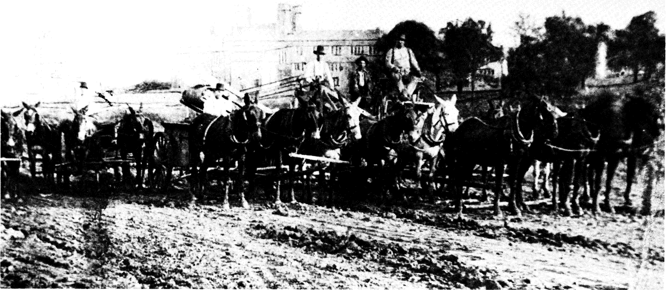
This is the type of equipment used for early road and railroad right-of-way construction (William H. Wignall).
