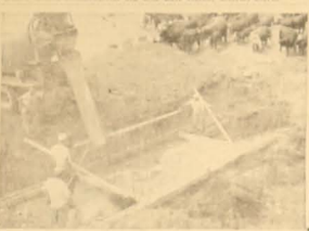
CONCRETE IS BEING POURED for the Dale Minger structure. It will be used with rock to form the dam.
