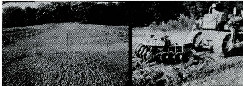
No grass was available on the demonstration farm for an outlet for the terraces. This ridge outlet was constructed, fertilized, and seeded to reed canary grass.
