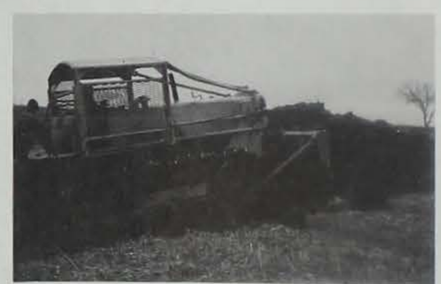
A dozer beginning work on push-up grassed backslope terrace construction on the Vernon Corrington farm near Washta.
