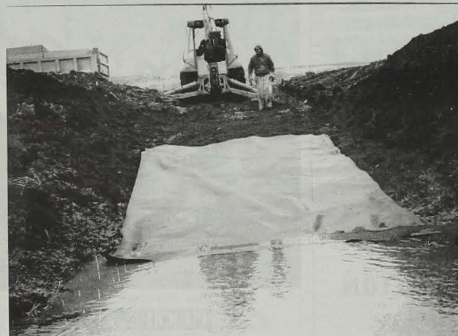
The above two photos show phases in the process of constructing a low water crossing on the Bernie Bolton farm
