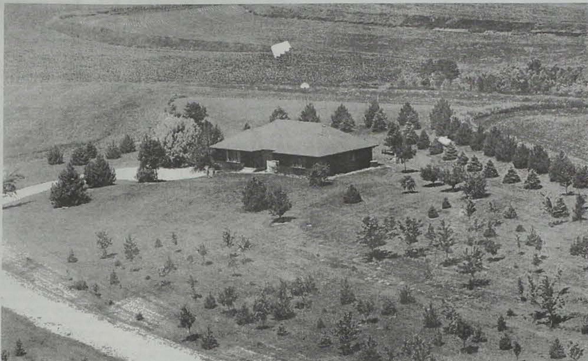
The Barry homestead, showing the larger trees which were planted before their house was built, and the smaller trees in the foreground which they added later.
