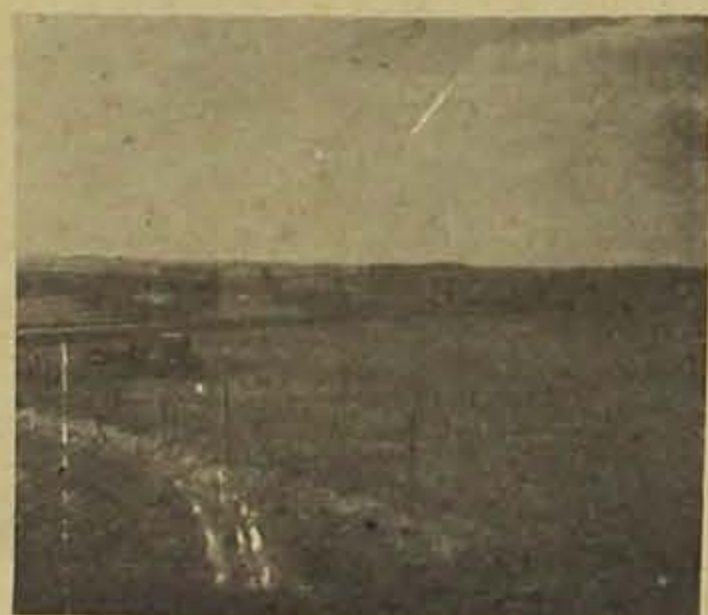
TERRACE SYSTEM ON THE MRS. FLORENCE McELROY FARM AT ELDORA.
