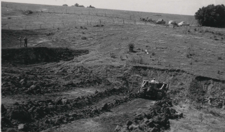
Olin Moshor - Ditch Filling - Aug. 50
