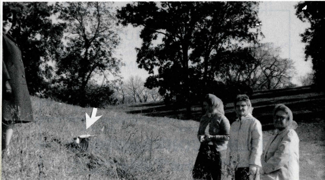
Newly built pond on the Gale Latham farm, two miles north-east of Montezuma. Note outlet pipe at point of arrow. Observers left to right: Auditor, Nellie Urich, Margaret Stemsrud, Katherine Yount and Marjorie Dieterich of the ASCS Office.
