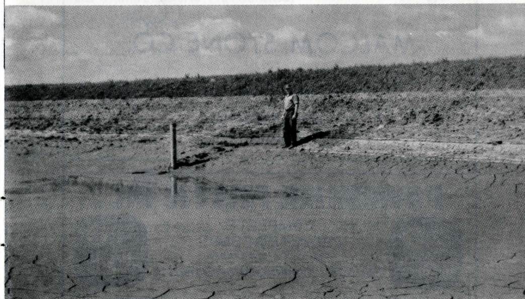
Flood retarding structure on Miles Clayton farm, 5 miles northwest of Brooklyn. The pond provides temporary storage until it can drain away through a tile.
