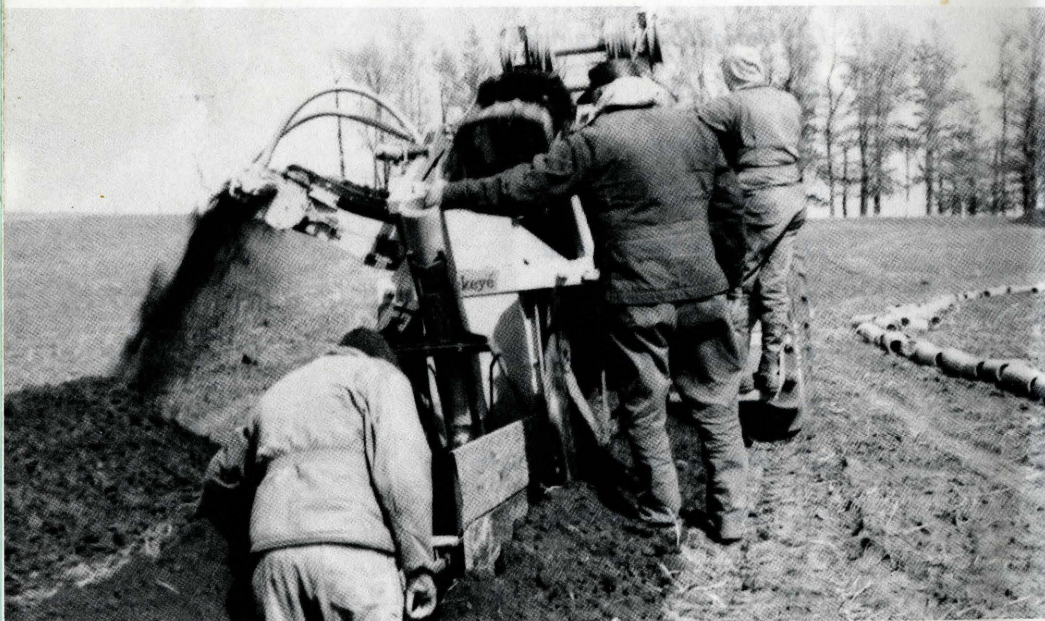
Tiling in early spring on John & Ferril Siehl farm, 4 miles north of Grinnell. During 1967 124 miles of tile was laid in the County.
