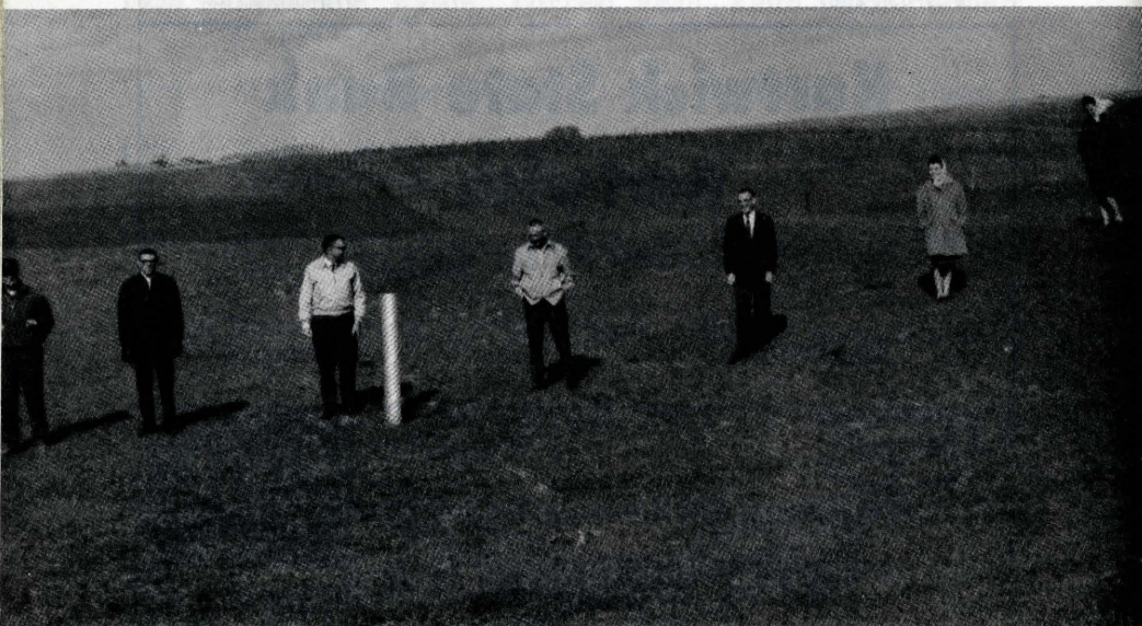
Personnel from the County ASCS inspect a flood retarding structure on the Ronald Bates farm, 5 miles north of Montezuma. Standing in the channel and on the dam, left to right Ronald Bates, Melvin Kasal, Gordon Braley, John Puls, Evan Johnston, Frances Schlesselman and Elizabeth Hewitt.
