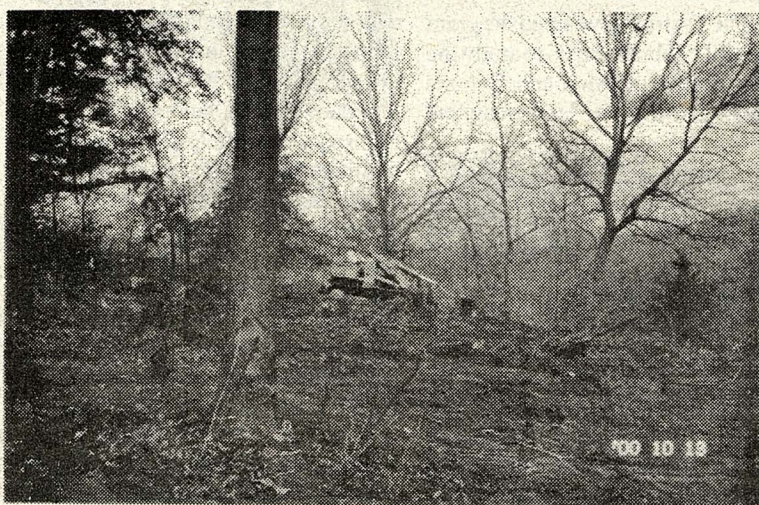
Site preparation being done on the Ralph Houg conservation farm, east of West Union.
