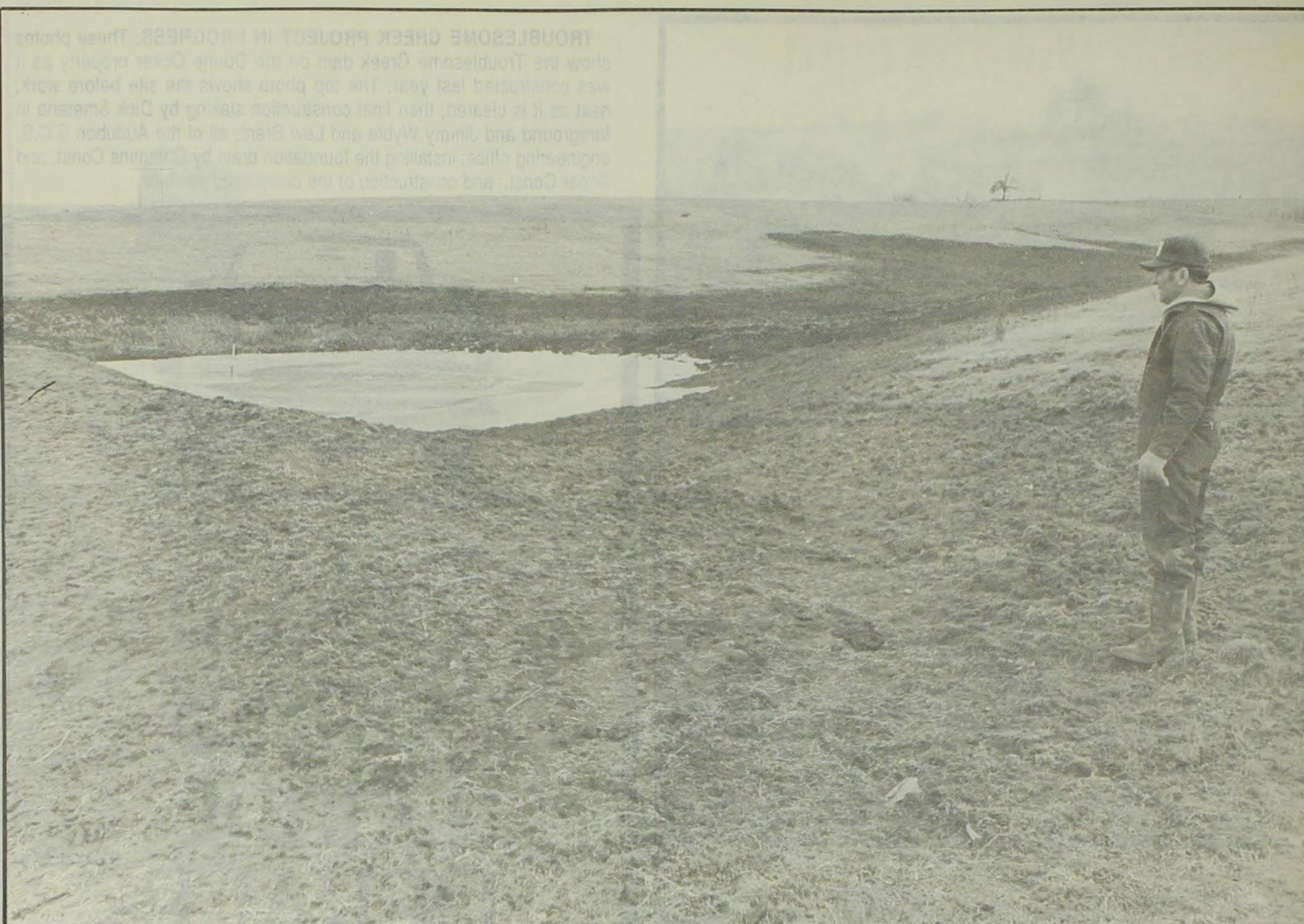
PRETTIER PICTURE. Bill Murphy, whose farm is north of Wiota, checks the filling progress of a new pond created when a dam was built on new ground he bought last year. The dam and pond cured an ugly gully
