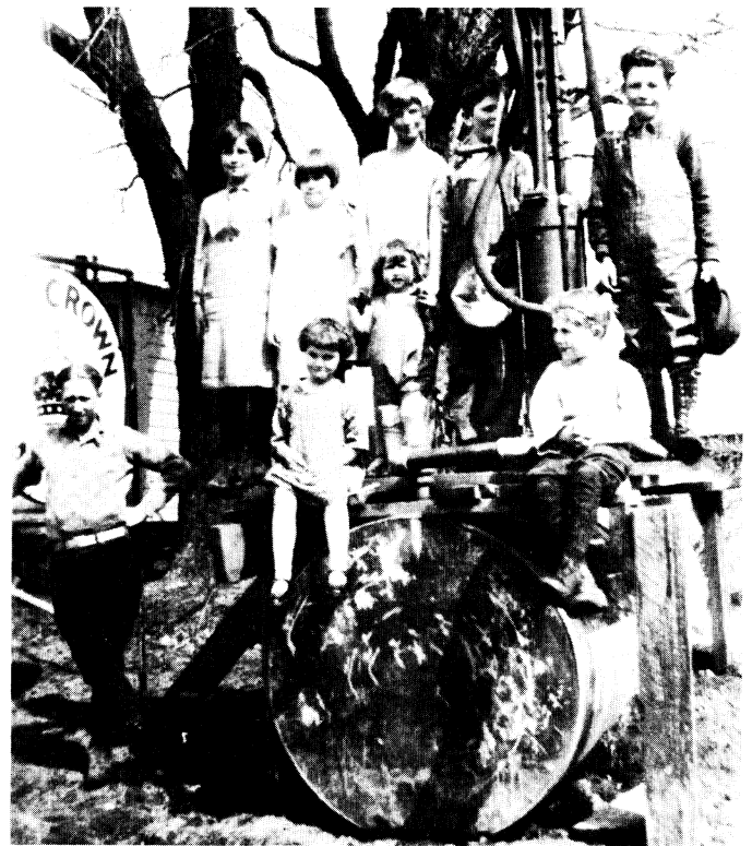
Eldridge children on gravel equipment in 1927.
