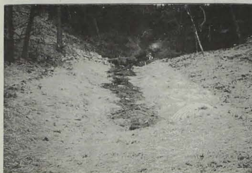
The same site with new installation in place, November, 1998.
