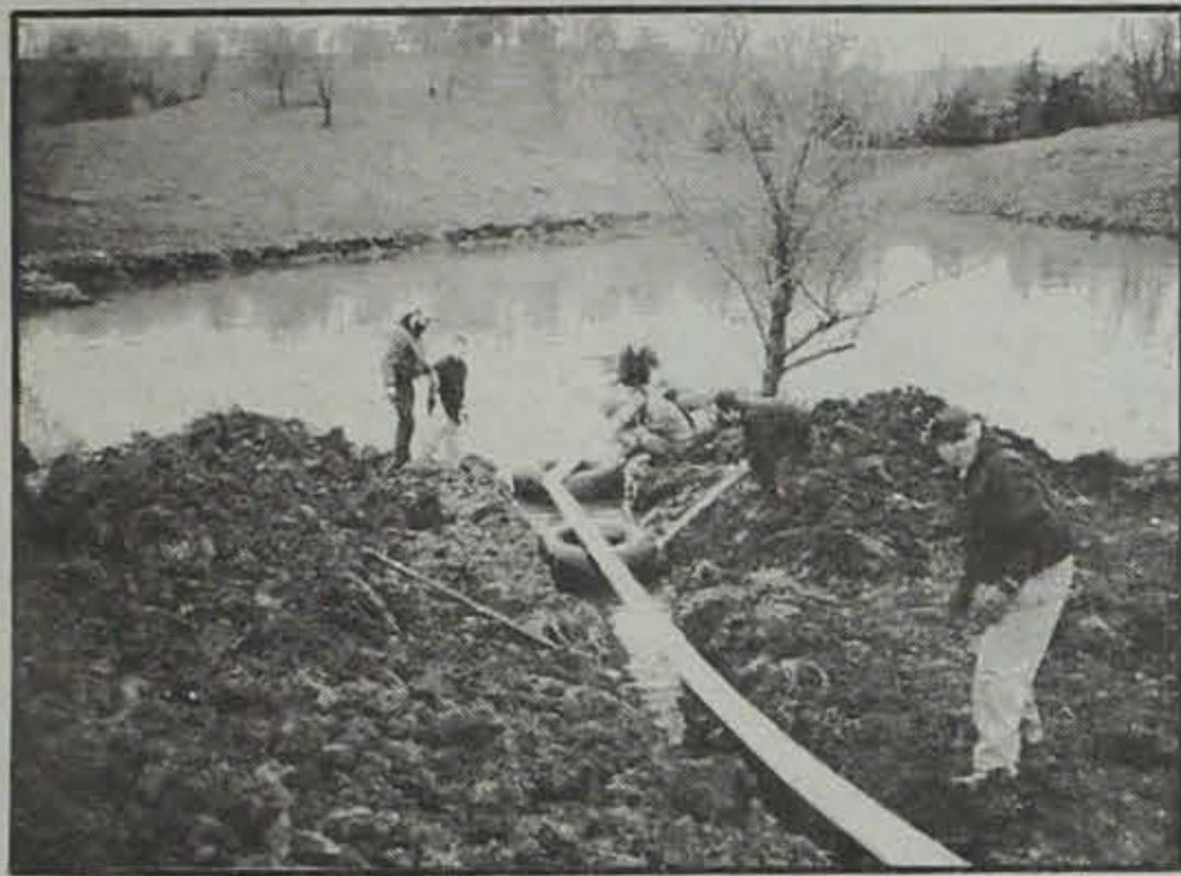
It takes manpower to put in the dry fire hydrant on the the Dean Rush farm in Southeast Pott county.
