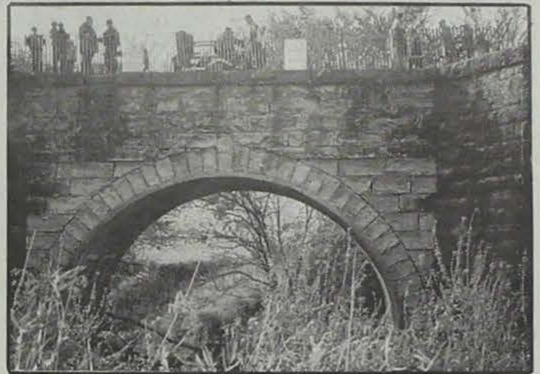
This historic old arch, for which the nature trail was named, has been nominated for inclusion in the National Register of Historic Places.
