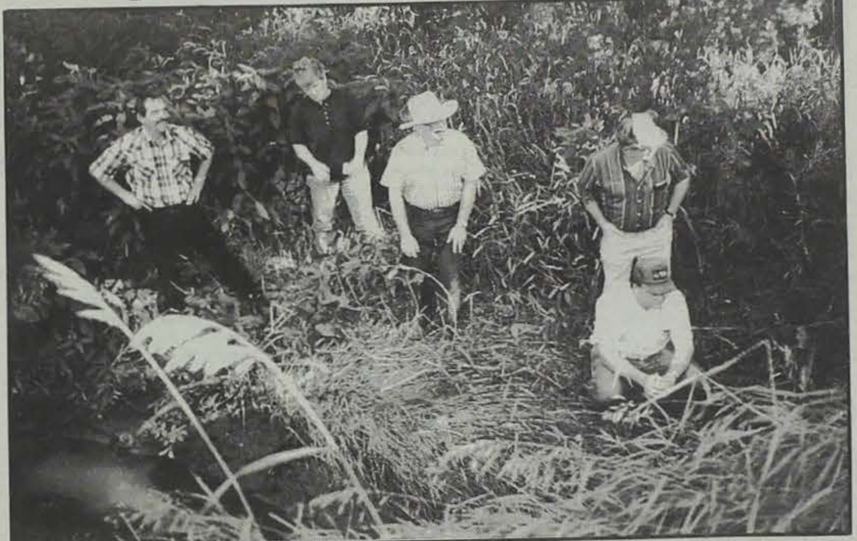
Russ Kurth, commissioners Anita Metter and Dwight Mills, Charles Carrigan and Engineer Mark McCurdy (kneeling) examine damage at the site in 1977.
