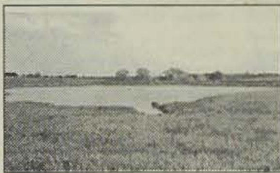
Grade control pond constructed in 1994 on the Bob Upfield farm.
