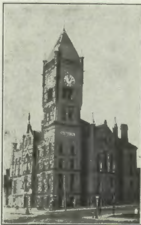
WAPELLO COUNTY COURT HOUSE
