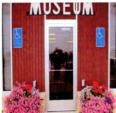
Louisa County Historical Society replaced two doors
