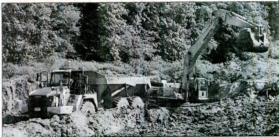
Removing silt from west side of the beach area at Lake Geode.
