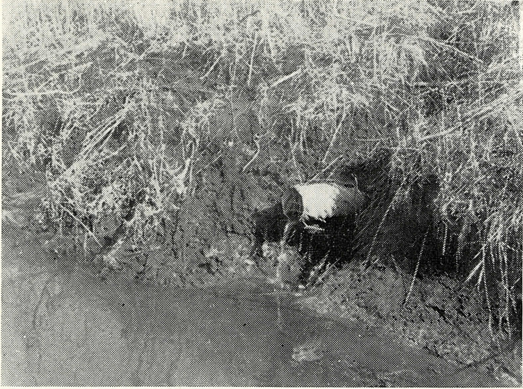
Need for tile drainage was critical on most Cedar county farms last year. This 16 foot corrugated tube, with wires through it to keep small animals out, will protect the tile outlet on Verda Wilson's farm, Center township.
