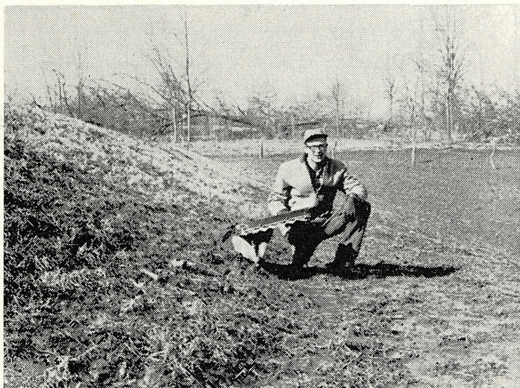
Allan Ball observing hooded inlet on his gully control structure.
