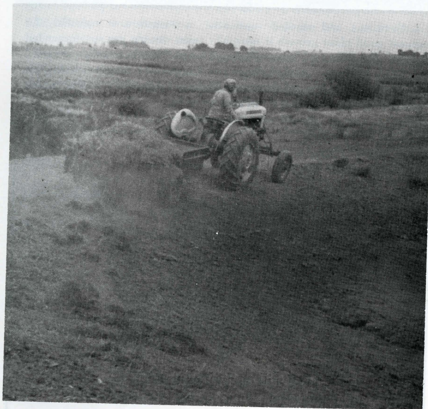
Picture shows Al Meacham, Cooperator, on tractor spreading straw over recently built structure after has been seeded. Al lives in Washington Township, Section 4, 4 miles south of Grinnell.
