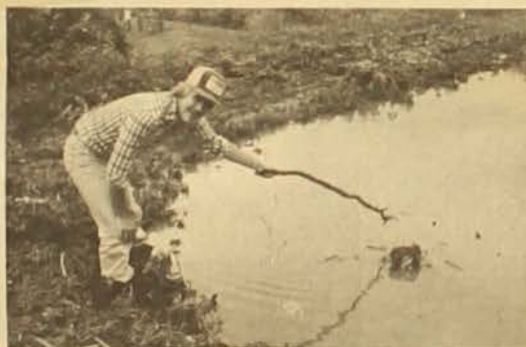
Kevin McCall, Soil Conservation Student and Trainee, clears debris from the tile intake terrace that helps prevent silt from entering East Lake.
