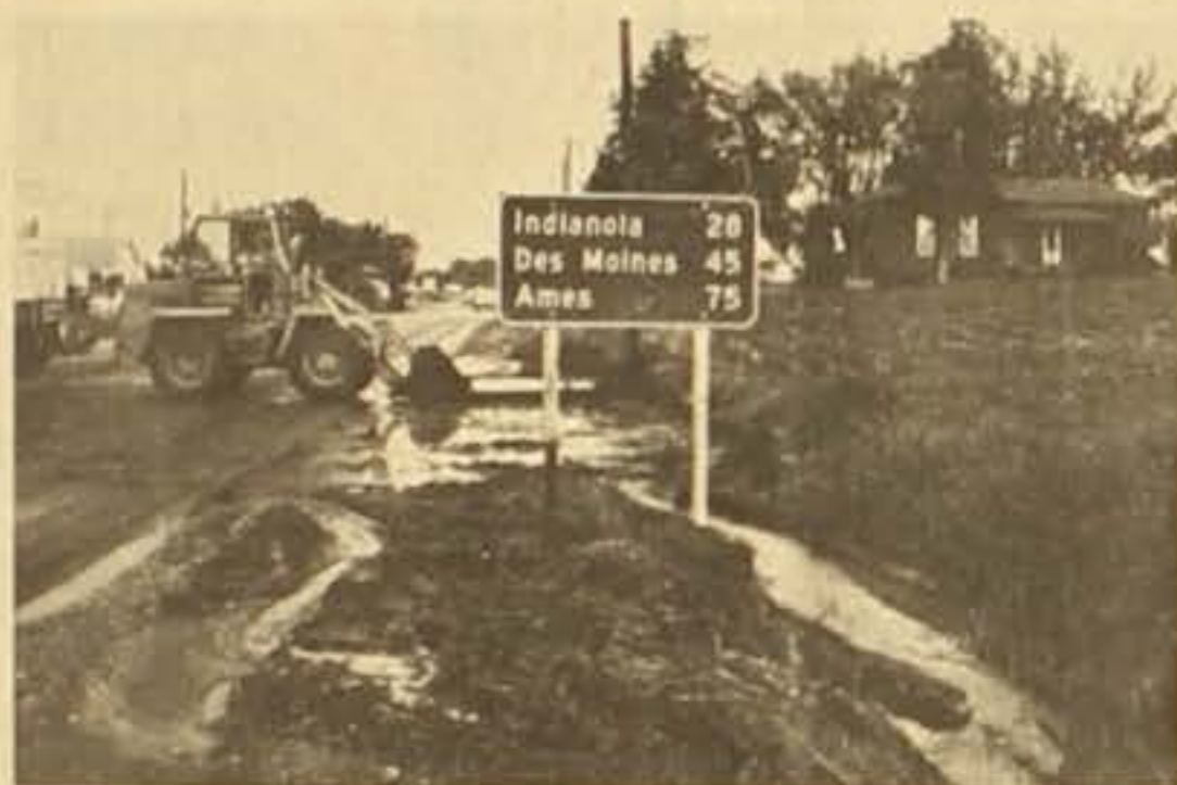
Iowa Dept. of Transportation crews are removing some of "Iowa's Best" topsoil along highway 69 just north of Osceola near the U.S.D.A. building. Keith Edwards, District Conservationist says this points out that soil erosion is one of the major problems of American Agriculture for both the farm and non-farm citizen. The cost of soil erosion is real, sizeable on a short-term basis, and enormous in the long run. The loss of an inch of this soil ultimately reduces crop production from 300 to 1,000 years.
