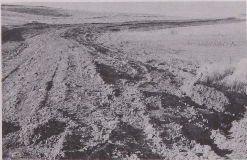
Diversion terrace constructed on the Ward Handorf farm located in the Union Grove Lake watershed area. This terrace was constructed in the fall of 1969.
