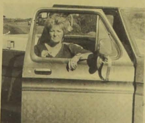
Joanne Welton operates the fuel truck to supply the heavy equipment.
