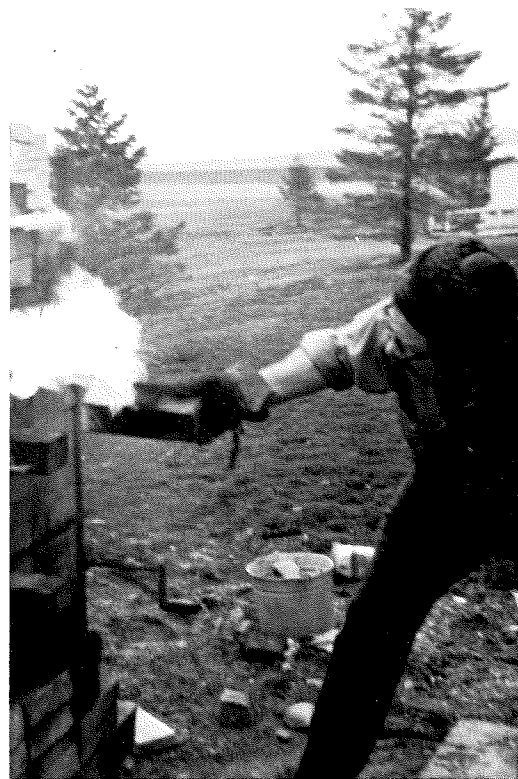
"It really works", a fact demonstrated by Mr. Mullen. The kiln appears to have a fiery temperament.
