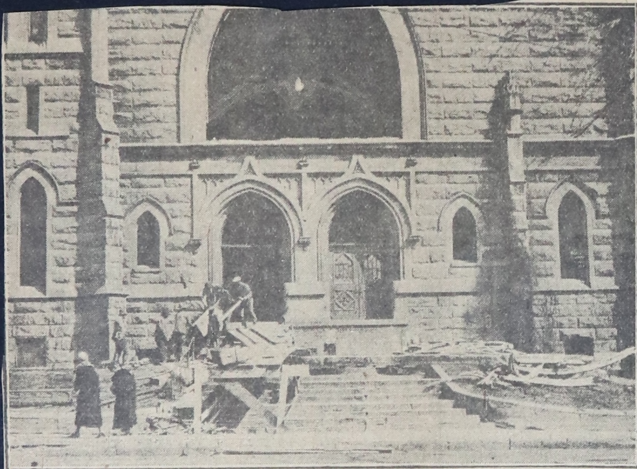
A BIT PATHETIC. The passing of an old church is not without its pathos, even when it is to be succeeded by a magnificent new one. There are some heartaches incident to this work of destruction on the old Plymouth Congregational building at Eighth and Pleasant streets. —Evening Tribune-News Photo.
