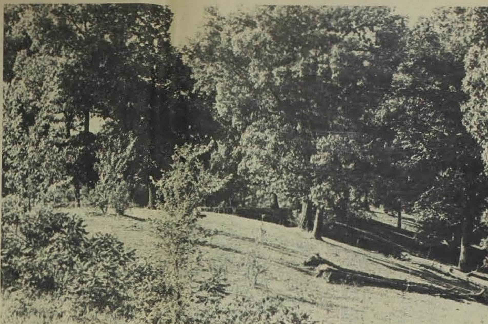
Caution: clearing under way
