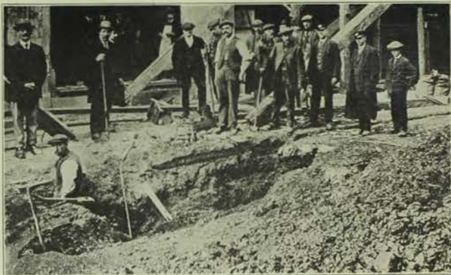
Clearing Away the Marks of an Air Raid
