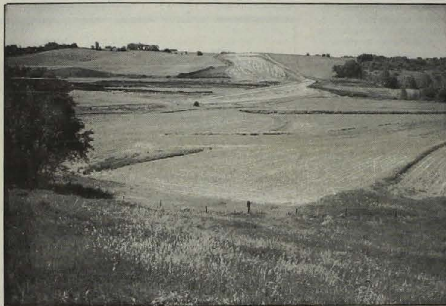
In the center background of this scene, taken early in the construction stage, may be seen the "borrow" area. Dirt taken from the hillside was used to fill the gully and build the dam.
