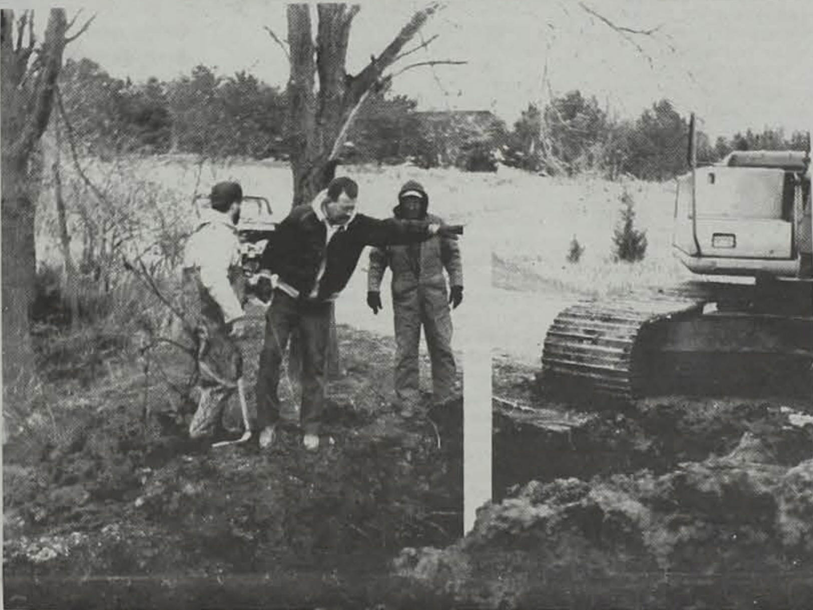
East Pottawattamie has two dry hydrants, and plans to install several more. The installation process is the same as shown in the above photo, where a suction pipe and strainer are being inserted in Willow Lake near Woodbine,.
