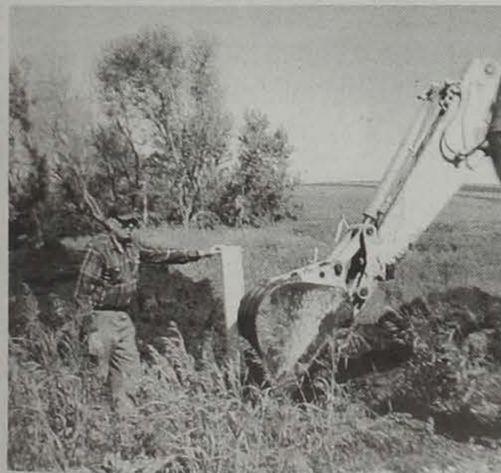
Bruce Damgaard, volunteer dry fire hydrant coordinator, steadies the pipe as the trench is being backfilled at an East Pott. site.
