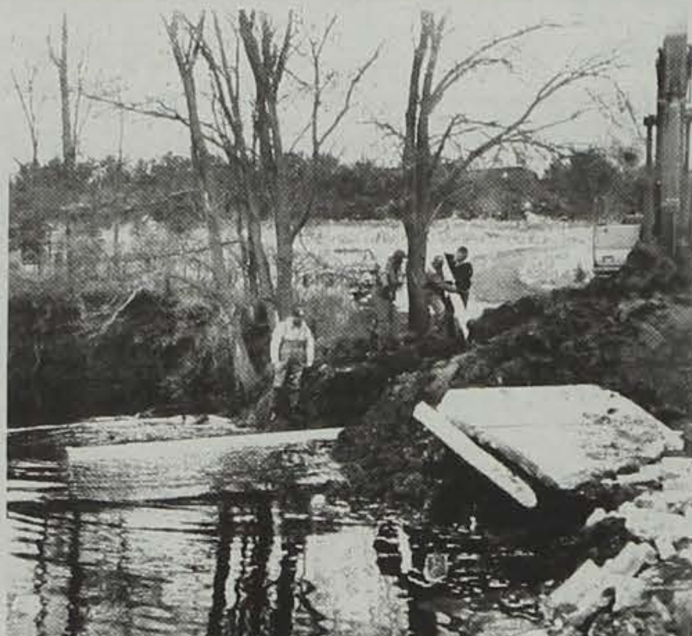
Rural Fire Hydrant
