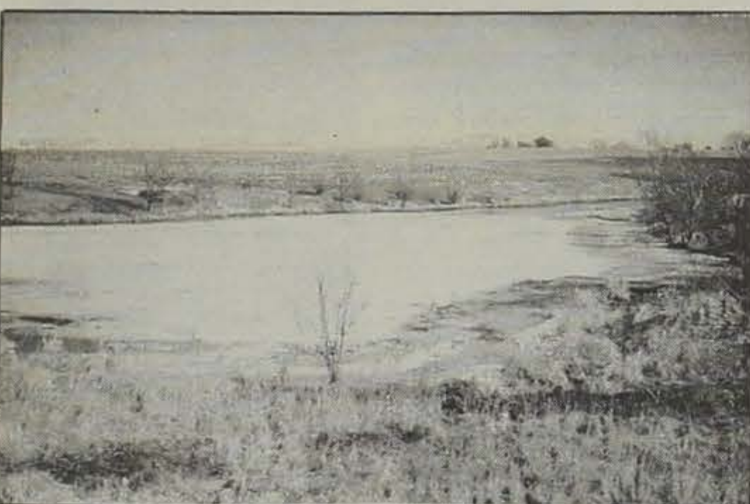
This structure in Harmony Watershed near Logan is still serving to stabilize road L 34. The gully in the background was once larger and deeper.
