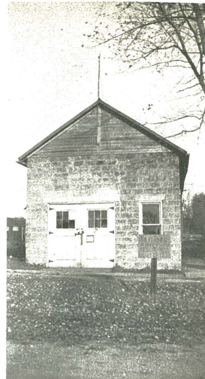
Town Hall and Fire Dept.
